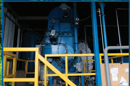
YORK & SHIPLEY 800 HP WOOD OR GAS FIRED PACKAGE BOILER
