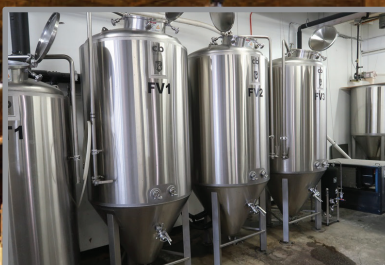
(3) PORTLAND KETTLE WORKS 10 BBL FERMENTATION TANKS
