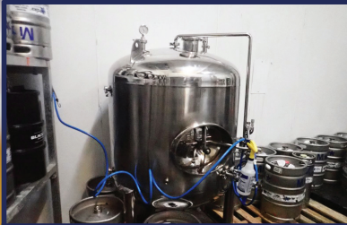
5 BBL S/S JACKETED BRITE TANK
