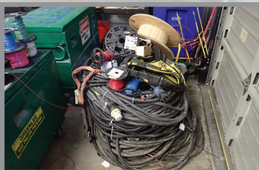
TEMP POWER WIRE
